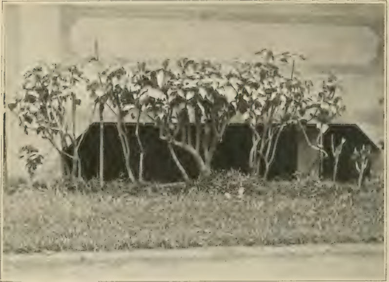
Figure 1. —Base of Caluan Hospital showing height above ground.
