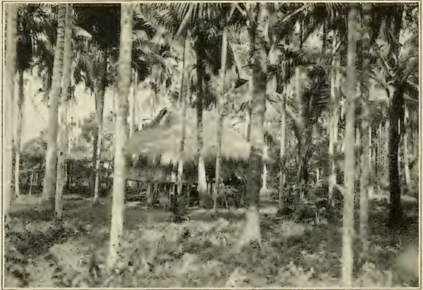
Figure 1.—Filipino rural house well shaded by coconut trees. A. minimus is breeding in large numbers about 30 meters beyond this house. On one occasion adults were caught in the daytime inside this house.
