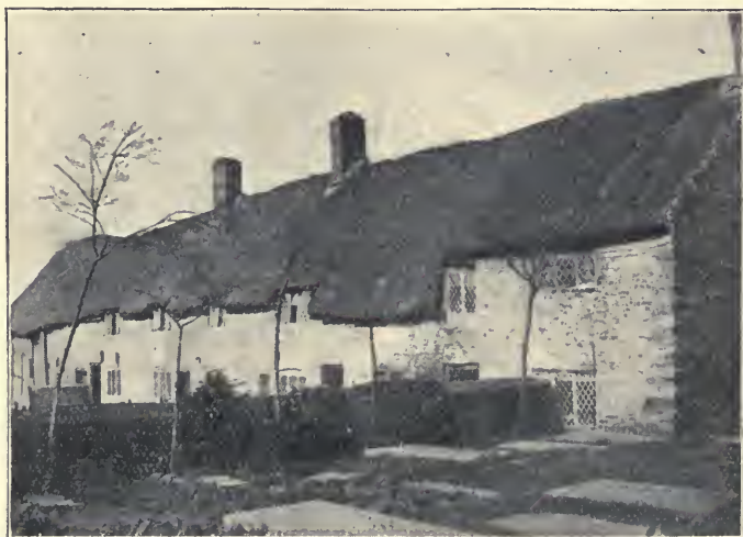
COTTAGES AT DENTON CHAPEL.
